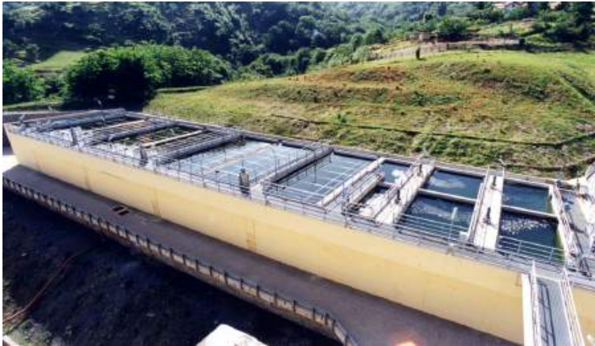
One of the gathering basins used for treating water.
