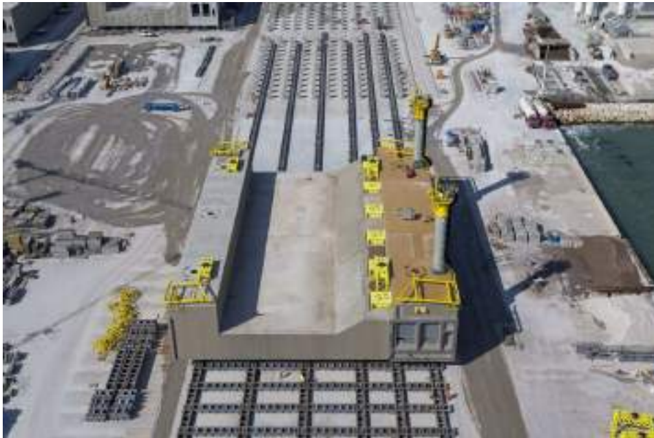
3. A threshold caisson
