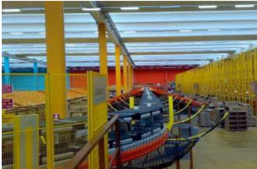
The Thun Logistics center's plant production floor completely managed by Movicon.
