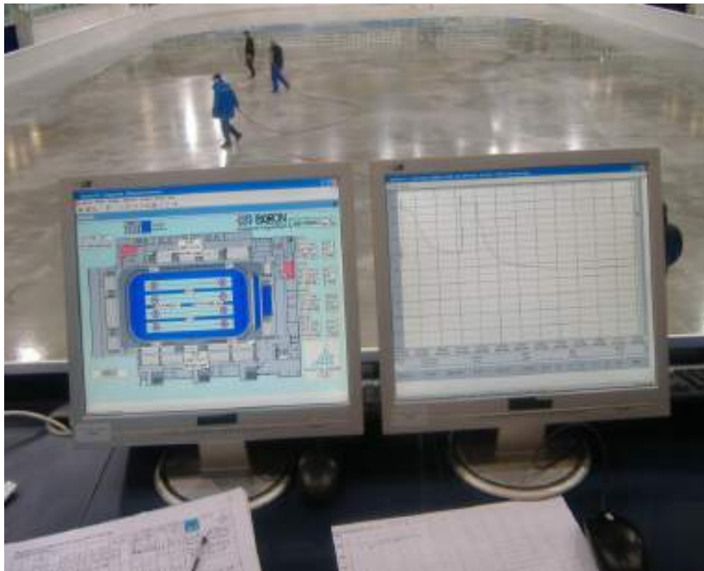
The Ice Rink Control Room, from where the operators manage the sport complex by using the Movicon supervision system.
